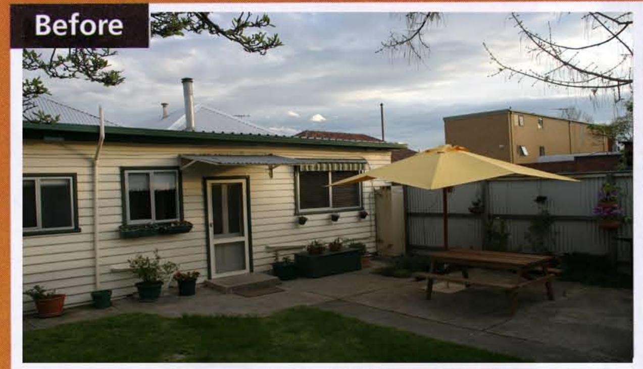
Left The untidy rear of the house before renovations.
